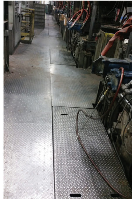
Row of molding machines before upgrading steel plates to safety mats
